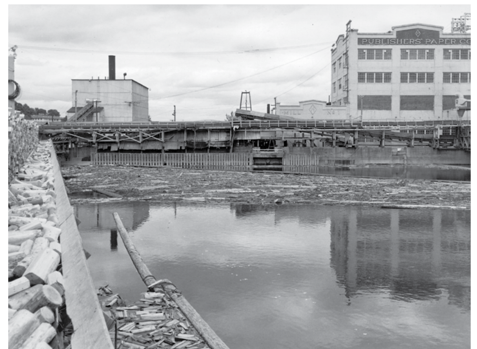
Hawley/Paper Machine No.1 Building is a significant visual and historic icon and occupies a prominent position on the Lagoon and at the south end of Main St.
