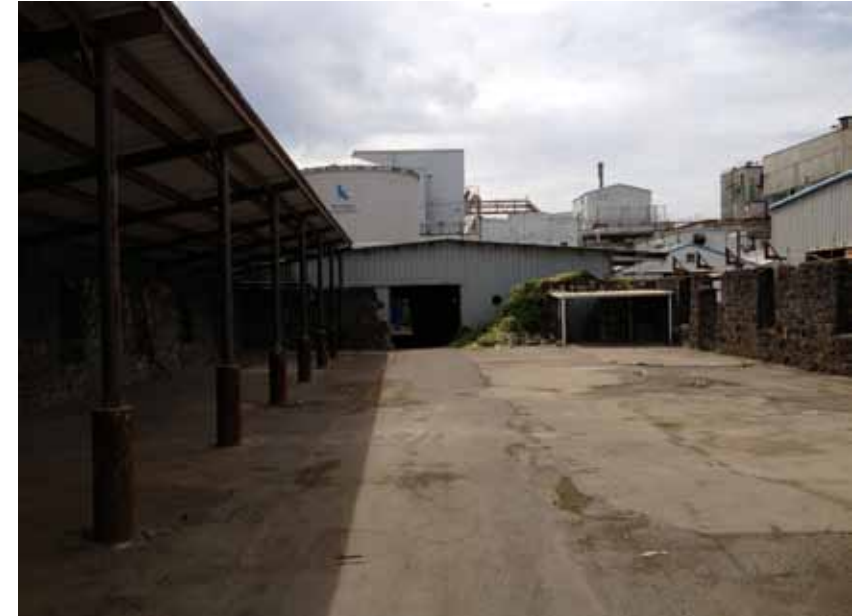
Exposed basalt foundations of demolished Woolen Mill.
