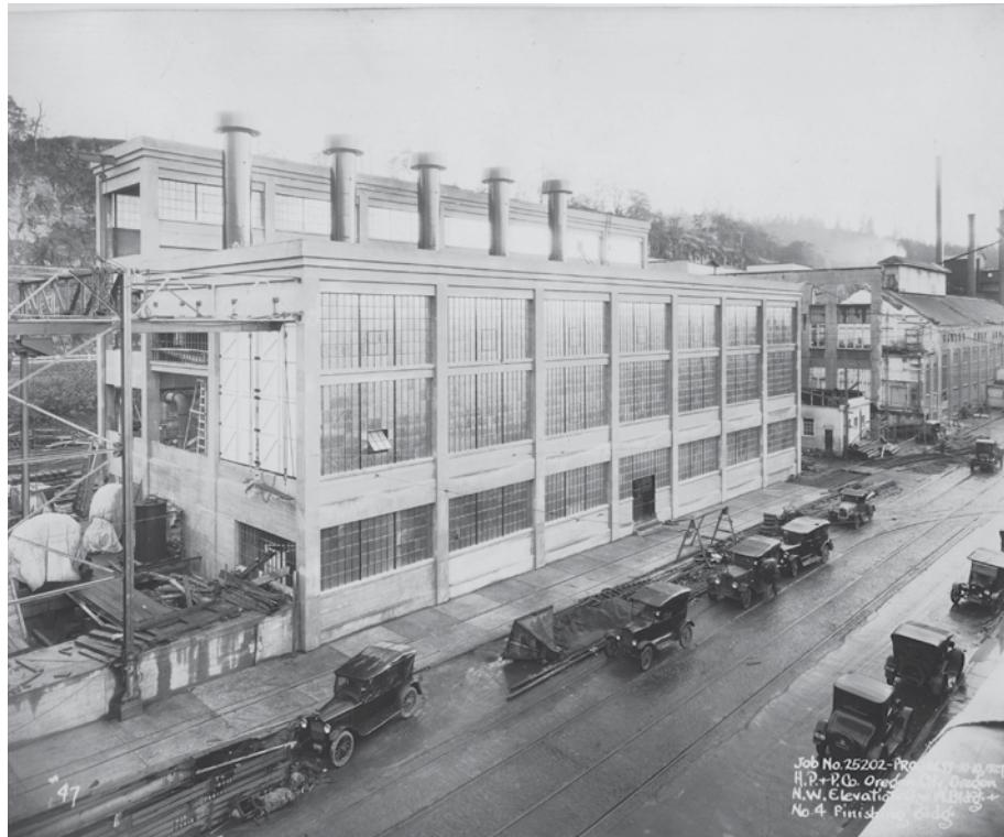
No. 4 Machine Building. Many of the buildings were designed with a very pure and rigid geometry that has been lost over a century of additions and renovations.
