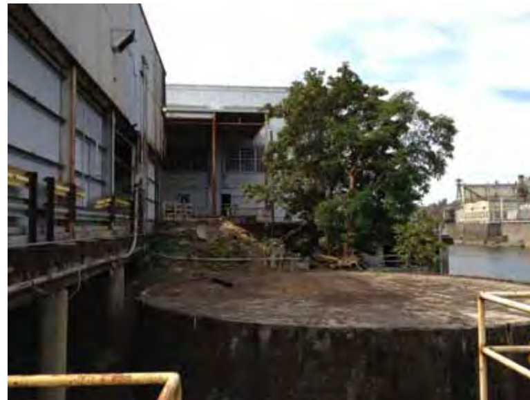
Concrete platforms overlooking the Willamette River. Repurposing options could include viewing decks.
